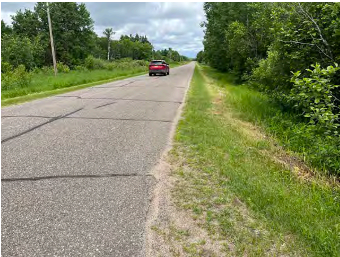
Looking north down 281 st Ave
