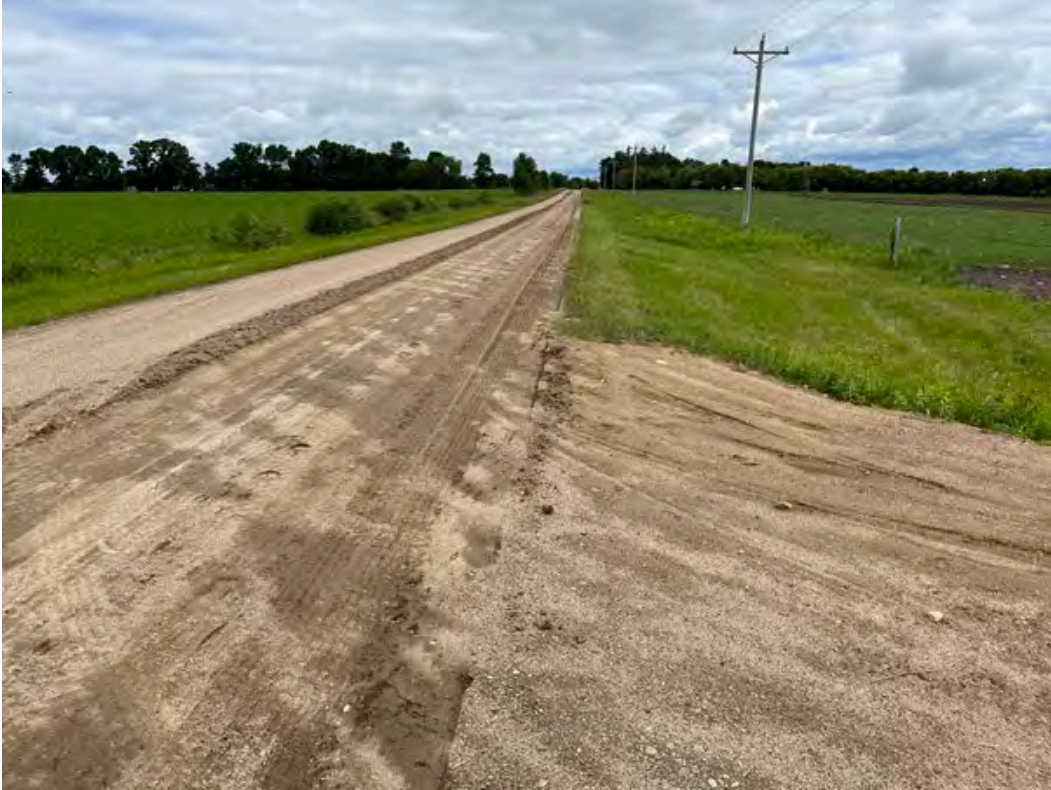
Looking north down 185 th Ave
