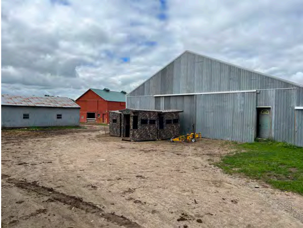
Looking southwest from center of the building site
